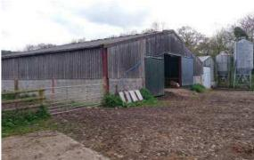
Steel-framed covered silo, 75' x 30'. Spaced boarding gale cladding with box profile side cladding above mass concrete wall.
